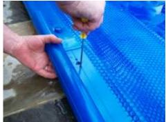
Using a screwdriver, go through the fixing holes to make a hole in the solar cover.
