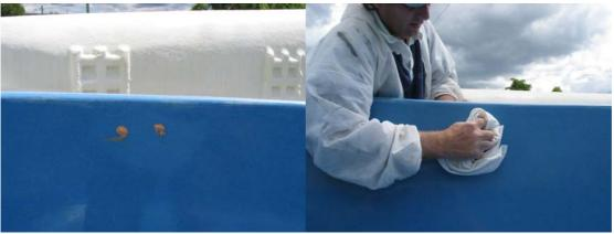
Once buffed, inspect to ensure good finish. Failing which, apply more cutting compound and buff.
