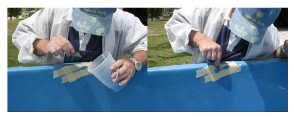
• Remove the masking tape and wait until the gelcoat has hardened. Depending upon the temperature the time to go hard will generally vary between 1 to 3 hours.
