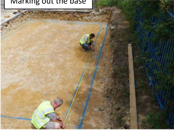
Marking out the base
